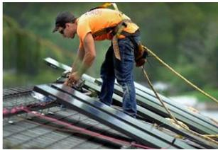
**Racking systems** attach the solar panels to the roof. Racks may be available in silver or black which is primarily based upon aesthetics and cost. So this is another important piece of equipment for your system but the actual racking system will be dictated by the panels selected.
